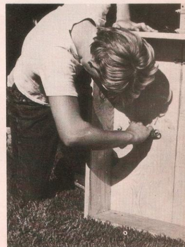
L. Bed of trailer is simply a sturdy box and care should be taken not to over-tighten bolts.
