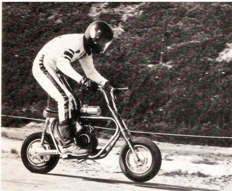
FINISHED - Complete with lightweight transplanted engine, the HPE Endura looks neat and nasty. Although front wheel could be lifted on dig-out, performance was effected by gearing.
